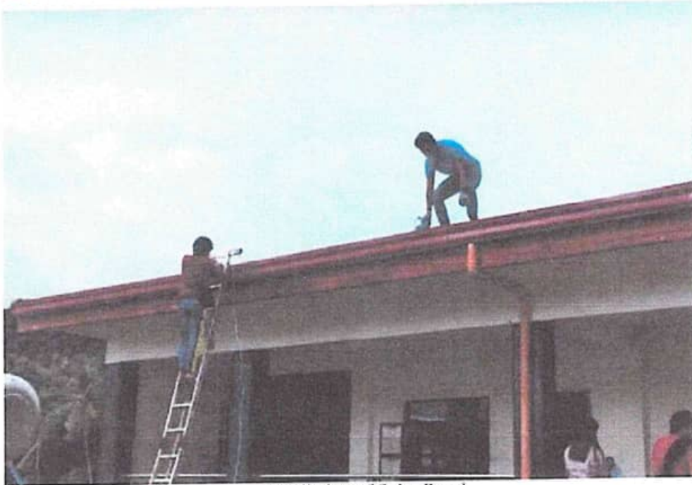
Installation of Solar Panel
